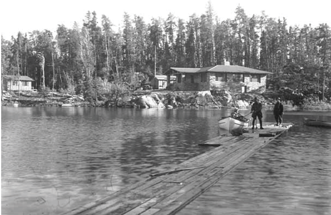
Figure 4- 20: HV#7, Historic View of Chik-Wauk lodge and surrounding area from across the bay, facing south, ca. 1936 (source: USFS)
