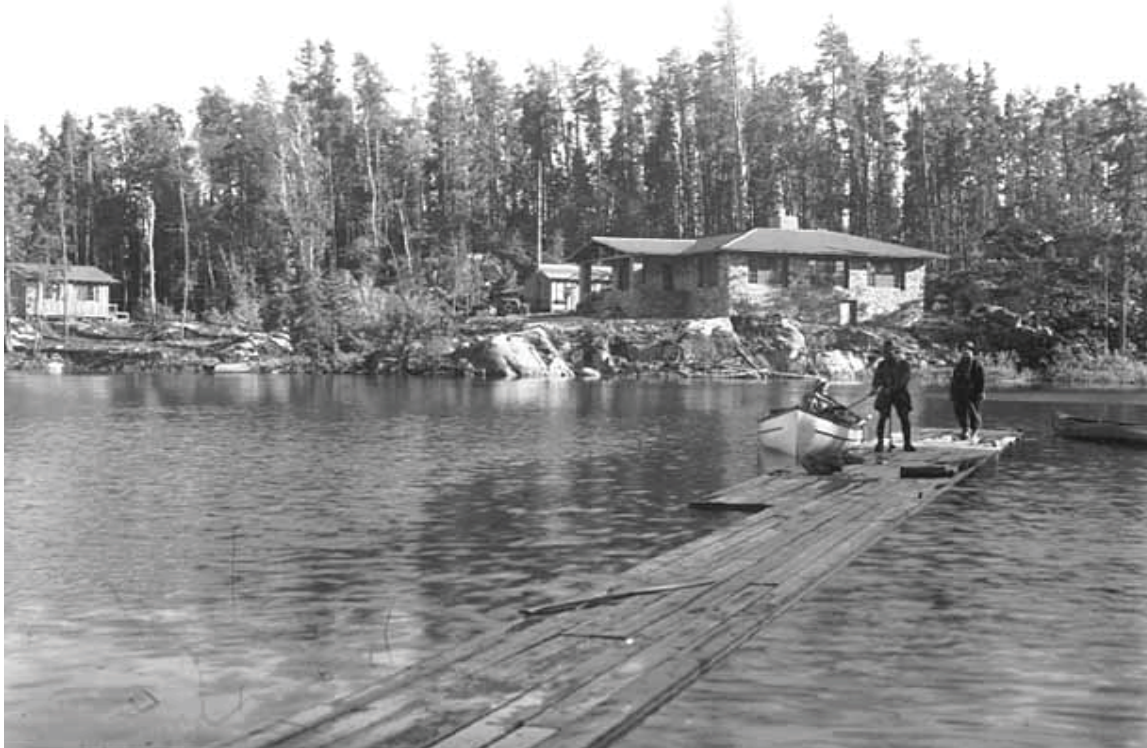
Figure 4- 20: HV#7, Historic View of Chik-Wauk lodge and surrounding area from across the bay, facing south, ca. 1936 (source: USFS)
