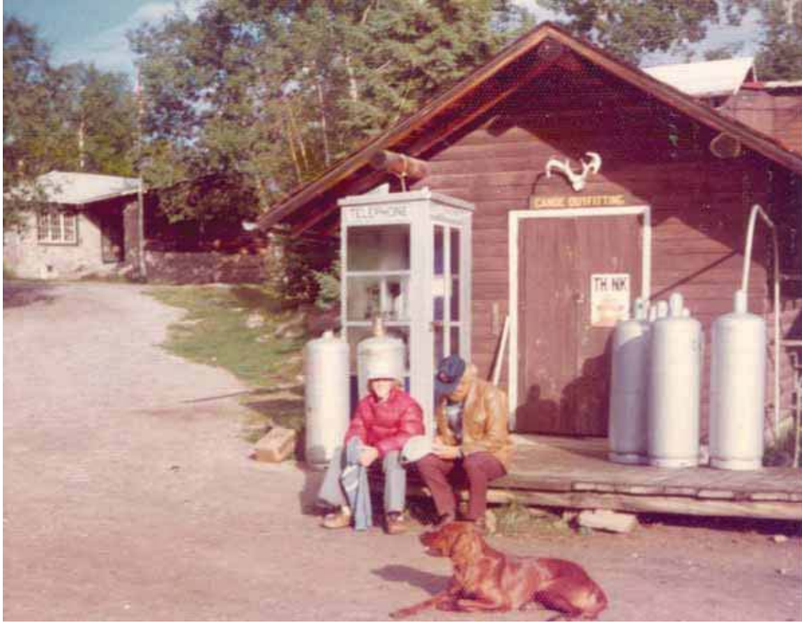
Figure 2- 41: Canoe Trip Outfitting Building, 1974 (source: C-W 188)
